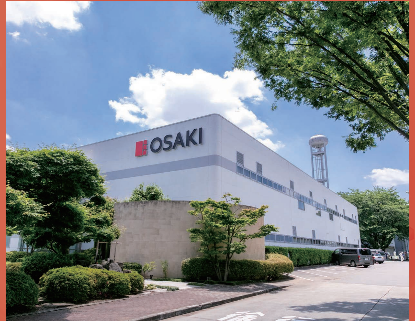
OSAKI ELECTRIC Saitama Factory
