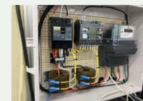
Meter board with local 5G
